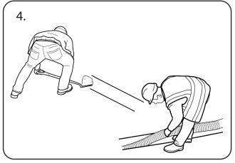
Excavate trenches and lay the required ducting. Between the Subsafe and power supply source and the Subsafe to the Orbital stem, thread the following cables: 1. Power supply from the source to the Subsafe 2. Circuit cabling from the Subsafe to the stem that requires the electricity supply.
